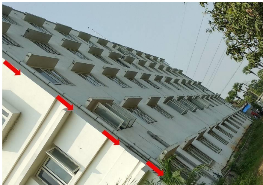
Pipe lines from roof top to recharge pits
