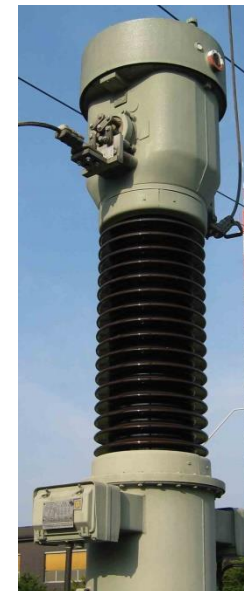
Fig. CT for operation on a 110 kV grid
